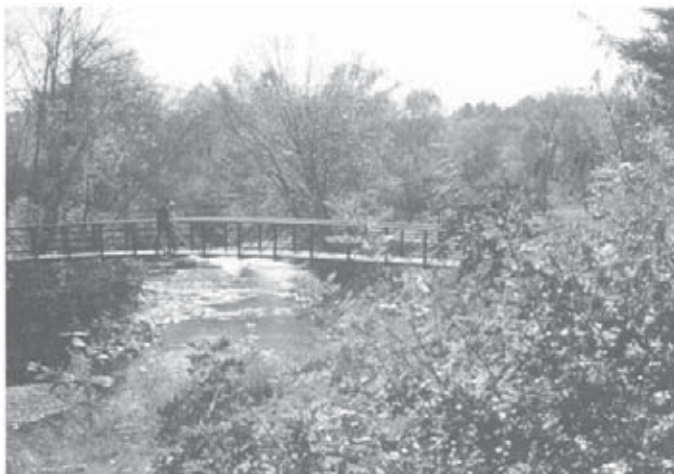
Fig. 27. The Stowe Recreation Path creates places of beauty for everyone to enjoy. Both the place and the process of creating it are dedicated to connecting private interests of abutting landholders to the public good.
